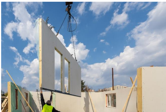
Timber frame cassette being craned into place
