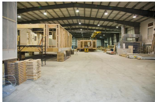
Pods being constructed under factory conditions
