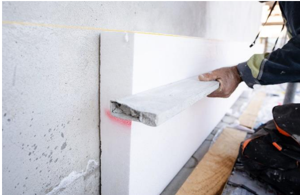
External insulation being applied
