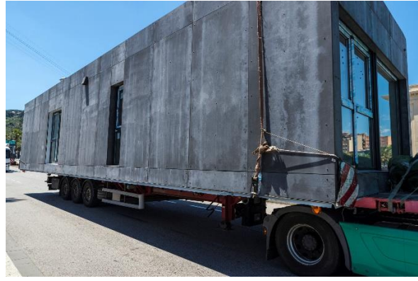
Concrete "pod" being delivered to site
