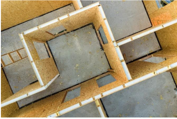
SIPs panels used in the structural walls
